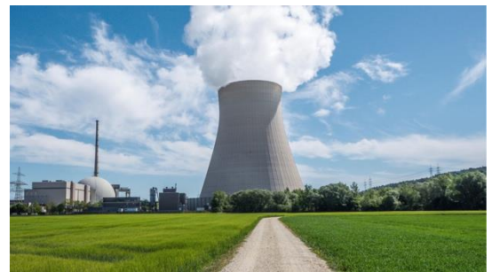
Figure 3: A Nuclear Power Station
